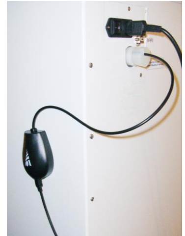
SAFE Sens® TrakPod™ installed in 200 l incubator Labo C201 via access port
